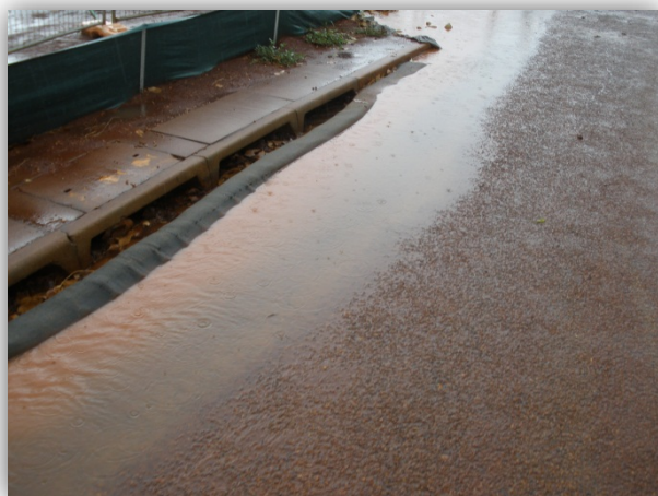
Effective side entry pit inlet protection
