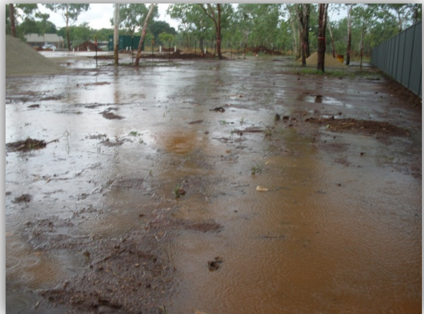
Construction site inaccessible after rain - lack of drainage and no diversion of upslope run-on.
