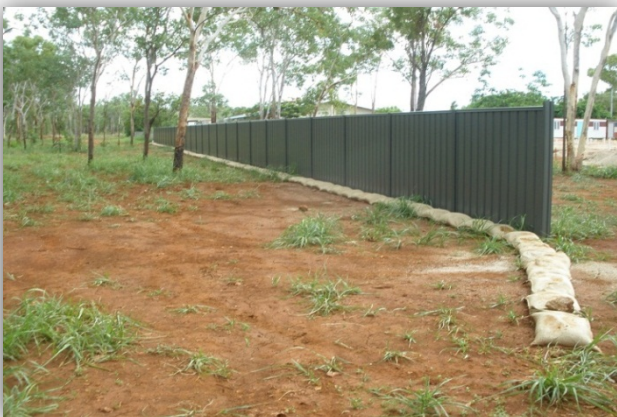
Upslope diversion bank (sand bags)
